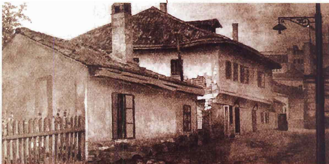
The subsequent building of the Higher School, nowadays the Museum of Vuk and Dositej
